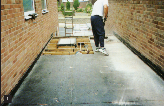
1 Fitted new plywood deck and then coated with bitumen primer.
