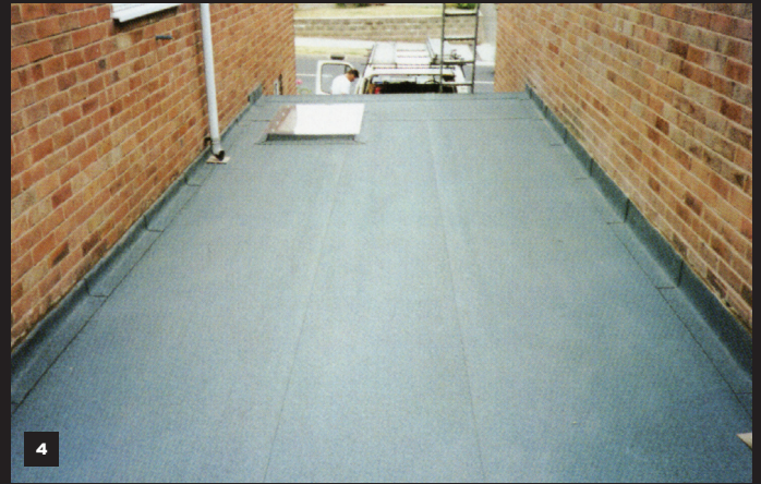
4 Final layer of Debotec polyester mineral finish capping sheet.
