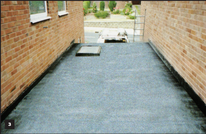
3 One layer of Debotec glass fibre underlay matt.
