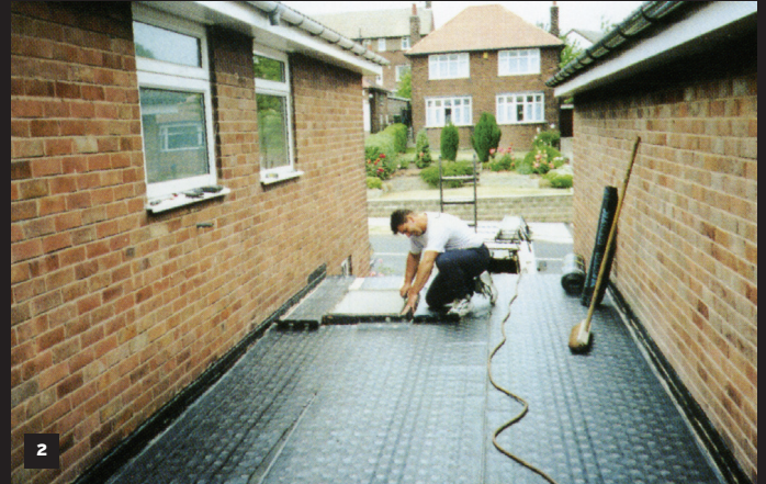
2 One layer of Debotec Debovent perforated layer.
