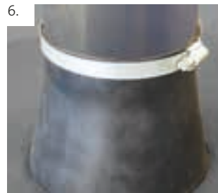
Finished outlet vent connection. «
