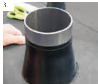
Pull the sleeve over the outlet vent.
