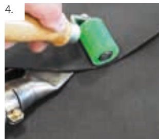
Weld to the roof surface.
