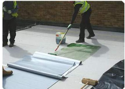
*Applying FF859 adhesive to the insulation*
