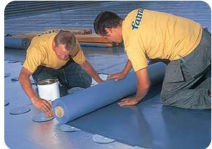
*Applying FF855 adhesive to the FF852 fixing discs*
