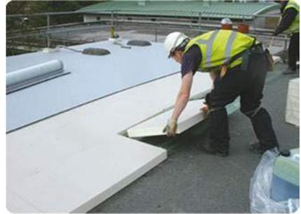
*Positioning the insulation boards*
