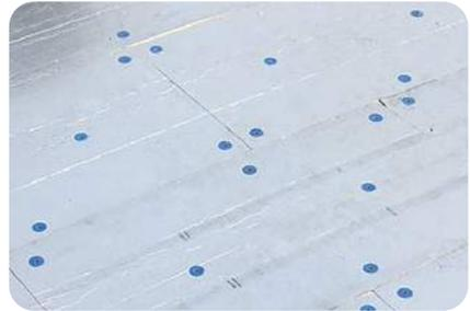
*Insulation secured with FR-75 tube washers*
