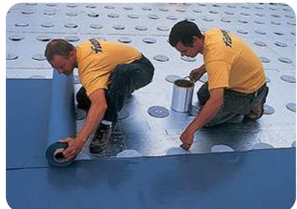
*Lining up and rolling out the membrane*
