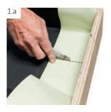
Cut the release film of the strip which is in contact with the stop end, across the height.
