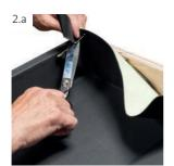
Cut halfway into the cone shape, parallel to the gutter edge, but slightly lower.
