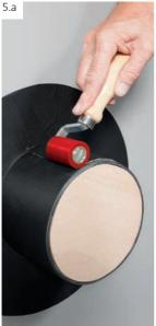
Press down the entire strip with a silicone pressure roller.
