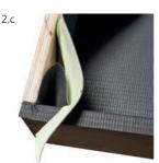
Now fold the cone shape inwards and apply pressure with the silicone roller, so as to maintain the shape of the folded corner.
