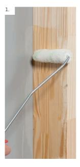
If necessary, prepare the surface completely with CCM primer. Apply it with a short-haired paint roller.
