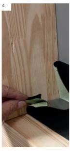
Remove half of the release film in the corner.
