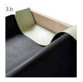
Double the strip at the cut release film and place it tightly against the stop end.
