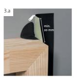
Fold the strip in half over the cutting lines and place it tightly in the corner. Remove the release film on one half of the strip, in parts.
