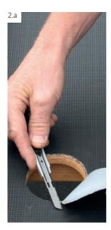
Cut off the EPDM at the opening of the rainwater outlet.
