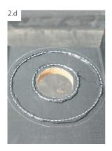
Apply HERTALAN® KS 96 sealant on the surface. Apply the KS 96 around the opening and at approx. 20 mm within the delineation.
