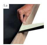
Start from the corner, against the stop end and remove the film in parts.
