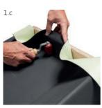
Press down the part without release film with a silicone roller against the stop end.
