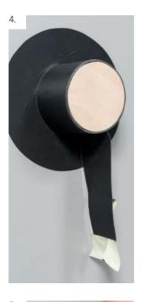
The width of the strip is a minimum of 100 mm. Cut the release film across the width in the middle of the strip. Adhere the strip, starting from the centre, to the passage.
