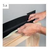
Fold the strip in half over the cutting lines and place it tightly in the corner. Remove the release film on one half of the strip, in parts. Press down with the silicone pressure roller.
