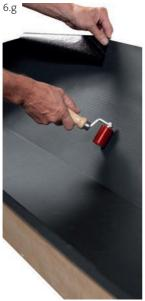
Finally, apply the strip upward in the same manner and press it down well with a silicone pressure roller.
