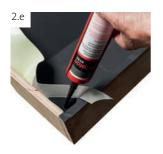
Apply HERTALAN® KS 96 between the two EPDM membranes (not too much) and push it firmly. Press it again when the corners have completely adhered.
