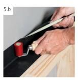
Remove the release film from the 2nd part starting in the middle. First press it down in the edge with the brass pressure roller and then do the level surface with the silicone pressure roller.
