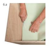
Fold the strip in half lengthwise, tightly in the edge. Cut the release film with the cutter knife
