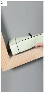
The release film on the underside strip is cut in the middle.
