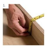
Measure the height and the thickness of the gutter edge plus 10 mm. In addition, measure the inner dimension of the box starting from the edge and add together all the dimensions. This is the "developed" width.
