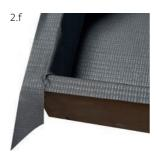
Now pull the last part of the strip over the gutter edge and roll it with the silicone pressure roller.
