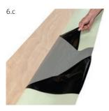
From the outer edge of the cut release film, pull the release film back to two sides. Do this well over the longitudinal cutting.
