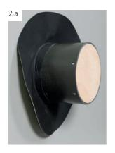
Cut the release film to the size of the diameter of the passage. Pull the sleeve over the passage. Make sure to apply it as low as possible.
