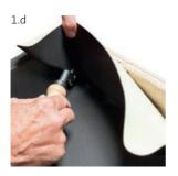
Fold into a cone shape in the corner. Press the strip tightly in the corner on both sides with the brass pressure roller.
