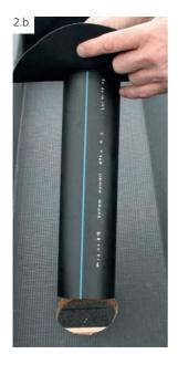
Place the PE pipe of the rainwater outlet in the opening.
