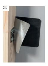
Fold the adhesive in half across the width and adhere it in the edge.
