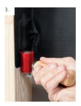
Then remove the release film from the inner side of the seal and roll with a silicone pressure roller. Repeat the process by removing the film from the 2nd part of the adhesive.
