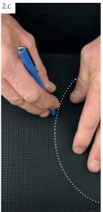
Line out the rainwater outlet on the surface.
