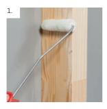
If necessary, prepare the surface completely with CCM primer. Apply it with a short-haired paint roller.
