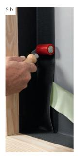
Remove half of the release film in the corner. Adhere this part to the vertical part. Then remove the release film from the upper part an adhere this to the vertical part as well. In such a way as to create a corner.
