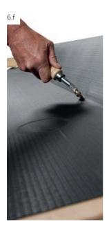
Lastly, press the EPDM down in the edge with the brass pressure roller. Then work the other side in the same way.
