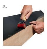
Press the strip down with the silicone pressure roller both against the gutter edge and on top of the gutter edge.
