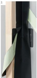
Fold the strip in half over the cutting lines and place it tightly in the corner.
