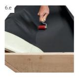
Text picture 4: Where the release film has been removed, press down the strip on the gutter base with the silicone pressure roller. Then remove another part of the release film and press down, repeating this procedure until the end of the strip.
