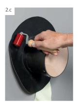
Press down the sleeve completely with the silicone pressure roller.
