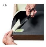
Fold the cone shape open. Where it has been already cut into, it can be cut into further exactly in the direction of the corner of the gutter, up to 5 mm before the corner.
