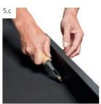
Press the strip down in the edge with the brass pressure roll.
