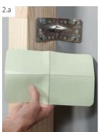
Cut out an adhesive measuring 80 mm more than the radius reach of the frame tie. Cut the release film crosswise with the cutter knife.
