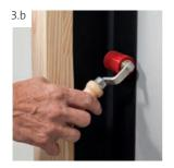
Press the strip with a silicone pressure roller. Repeat this procedure on the other side. When doing so, the edge must be pressed well with a brass pressure roller.
