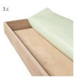
Fold the strip in half lengthwise. Measure the height and the thickness of the gutter edge here as well, plus 10 mm.
