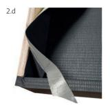
Carefully pull the release film from the cone shape. Push the first part against the gutter edge and then the rest.
