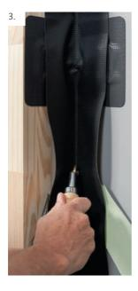
Press it down in the edge with the brass pressure roller and then the entire strip with the silicone pressure roller.
