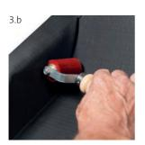
Let the strip of the gutter edge continue until the sloping part. Then apply the strip of the sloping part over it in a draining direction.
