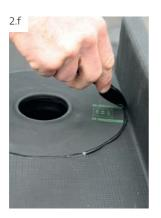
Remove the sealant line and smooth.
