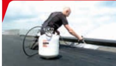
Product application without any need for naked flames is a requirement we have taken into consideration in our application techniques. The HERTALAN® seam joining method is implemented using hot-air technology and an EW joining edge that is ready-made in the factory. An emerging welding bead indicates an ideal and permanently safe seam connection. Alternatively, seams can also be adhered together.
