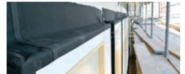
HERTALAN® is a plasticiser free material that is permanently resistant to UV rays, ozone and other natural atmospheric influences and is also extremely elastic within the temperature range of -45°C to +120°C. Thanks to its outstanding elasticity of up to 500%, it can be put to flexible use in various waterproofing situations. HERTALAN® withstands all tensile stresses that a flat roof is exposed to during the course of its normal life cycle.
