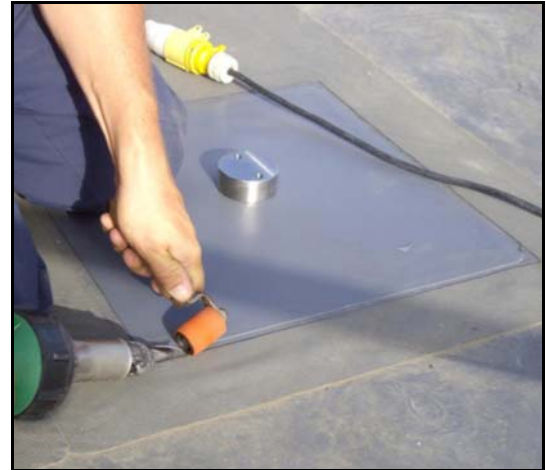
The membrane is heat welded to the surrounding roof field area
