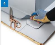
➤ Trim the corner to a rounded finish to overlap the first flashing.
