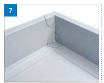
Weld the pre-formed corners (FF850 or FF851) to all 3 sides avoiding distorting the membranes by an excessive temperature build up.
