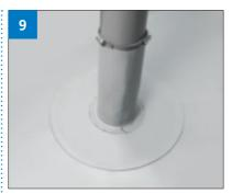
After the pipe detail has been completed pre-weld and final weld the collar to the area membrane.
