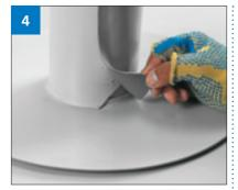
After tacking in position remove the sleeve from the pipe and cut the bottom 30mm of the sleeve lap at an angle to reduce thickness for stretching. Then replace back on to the pipe.
