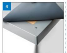
▶ The FF810 or FF804 can then be taken over the faceted metal and welded in line with the edge of the trim ensuring the cut edge of the trim is covered with the membrane.
