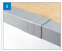
Lift the strap from under the metal up the face of the metal and weld to the face and top of the trim before finishing on the inside edge of the trim.
