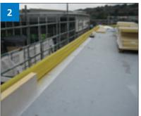
At up-stands and penetrations turn the vapour barrier up the vertical section to the height of the thickness of the insulation board which is going to be installed and seal to the vertical with butyl sealant tape.
