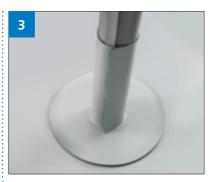
Cut a sleeve to a height of at least 200mm. Use a temporary length of FF804 to make the flashing oversized when wrapped around the pipe before tack welding the flashing around the pipe.
