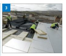
Loose lay the insulation board to a staggered bond pattern, following the manufacturer's instructions.
