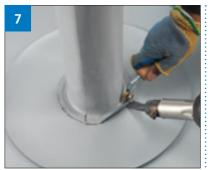
▶ Weld the 20mm flashing to the collar using a brass 'penny roller'.
