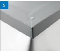
▶ If using a FF810 field sheet make sure the last line of fixing discs is 200mm from the edge of the roof then take the FF810 over the trim and weld flush with the outer edge.
