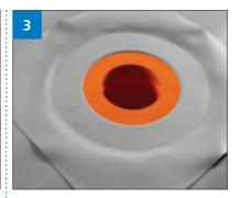
Lay the field membrane over the hole and cut to match. Then insert the rainwater outlet into the hole and push home ensuring that the outlet sits slightly below the level of the main roof.
