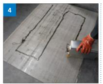
Apply Fatra polyurethane insulation adhesive FF867 to the substrate. The adhesive should be in 5mm beads at 300mm centres in the centre of the roof, 150mm beads for the first 2.4m in from all perimeters.
