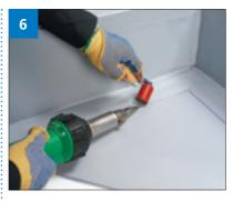
Weld up the vertical seam to the internal corner with a penny roller and then weld the horizontal flashing to the field sheet and to the top Fatrametal trim.
