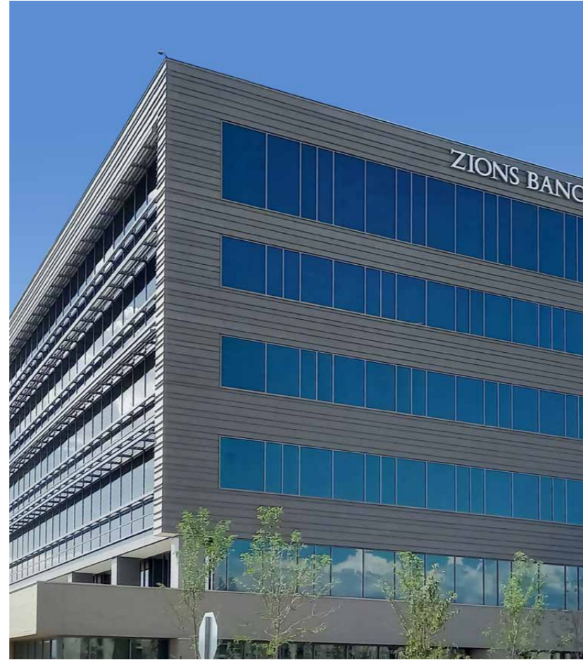
USA Midvale Office Building NedZink NEO Pro-Tec Standing Seam System
